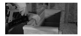
**08** Attach the front trim (D) with glue and nails. You should have an approximate  $\frac{1}{2}$ " overhang on the front and  $\frac{1}{2}$ " overhang on either end.
