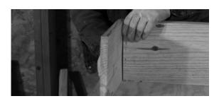
**05** Attach the front panel (A) to the side panels, keeping a ¼" overhang on each side.
