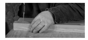
**04** Attach the side panels (C) to the back panel (B) with finish nails and glue, keeping the ends flush with the cleat and blocking.
