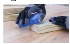
Ease any sharp edges with a medium grit sanding block. Apply preferred finish to the wood.
