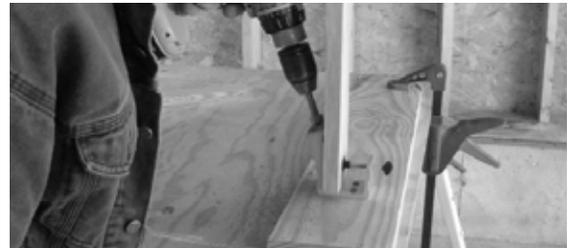
**04** Clamp the stock in place to its mating piece (spreading glue on the surfaces if desired), making sure to keep the edges and faces flush where needed. Gently drive screws through the drilled holes, stopping when the joint is drawn tight. Driving the screws too aggressively increases the chances of driving them right through the bottom of the drilled hole.
